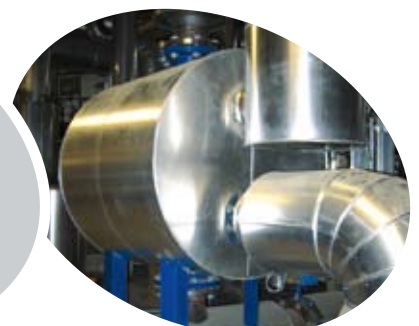
6 MW Process Water Heater PSHE 5LL – 134/1/1 Process water heated with thermal oil
